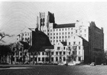
International House, University of Chicago, where many of the athletes were housed.
